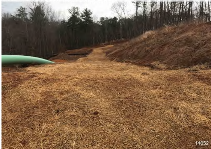
Figure 3: STA 14052+00 – Controls in place and functioning properly. Area stabilized with straw.
