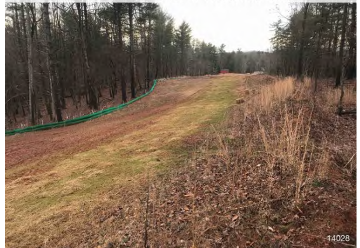
Figure 4: STA 14028+00 – Controls in place and functioning properly. Area stabilized with straw.
