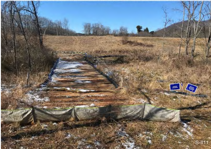
Figure 3: Stream S-II11 – Controls in place and functioning properly.
