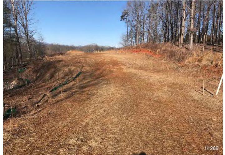
Figure 4: STA 14322+00 – Controls in place and functioning properly. Area stabilized with straw.
