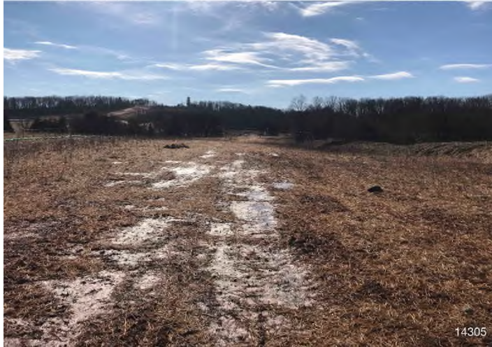
Figure 3: STA 14330+00 – Controls in place and functioning properly. Area stabilized with straw.
