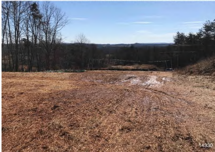
Figure 3: STA 14330+00 – Controls in place and functioning properly. Area stabilized with straw.
