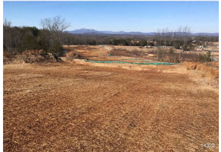
Figure 4: STA 14322+00 – Controls in place and functioning properly. Area stabilized with straw.
