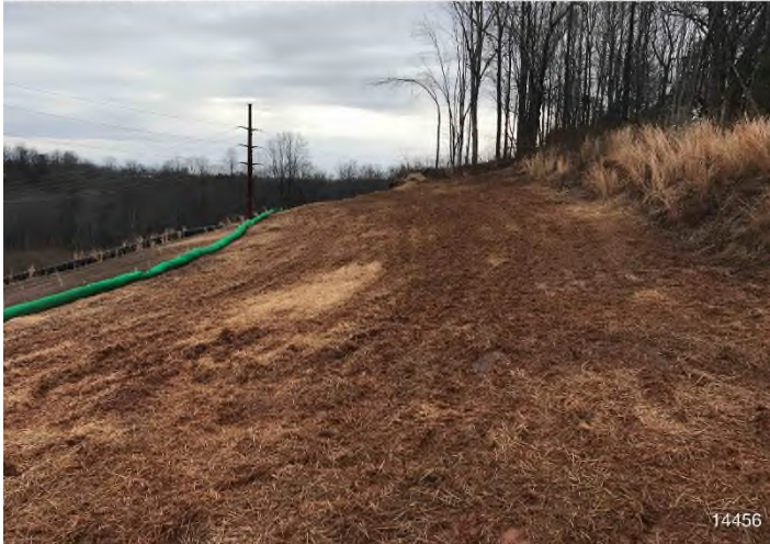
Figure 3: STA 14526+00 – Controls in place and functioning properly. Area stabilized with straw.
