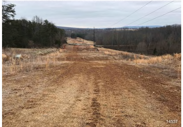
Figure 4: STA 14537+00 – Controls in place and functioning properly. Area stabilized with straw.
