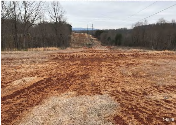
Figure 3: STA 14526+00 – Controls in place and functioning properly. Area stabilized with straw.
