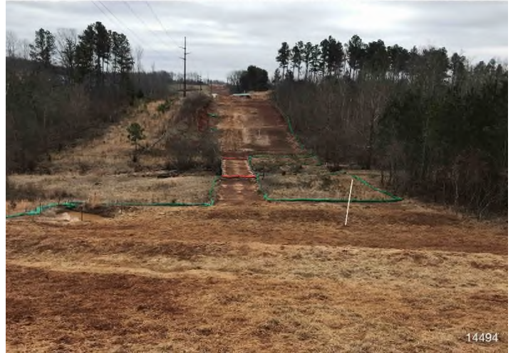
Figure 4: STA 14537+00 – Controls in place and functioning properly. Area stabilized with straw.
