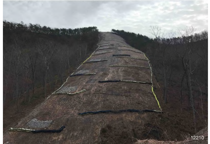
Figure 2: STA 12210+00 – Controls in place and functioning properly. Area stabilized with straw and erosion matting. BRG: 91°E (T) LAT: 37.253189 LON: -80.253902 ±334ft ALT: 1437ft
