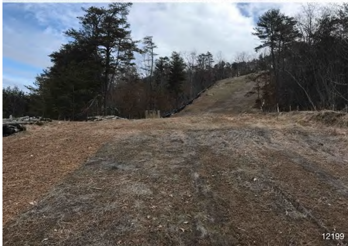
Figure 3: STA 12199+00 – Controls in place and functioning properly. Area stabilized with straw and erosion matting. BRG: 36°NE (T) LAT: 37.245846 LON: -80.258165 ±7129ft ALT: 1378ft
