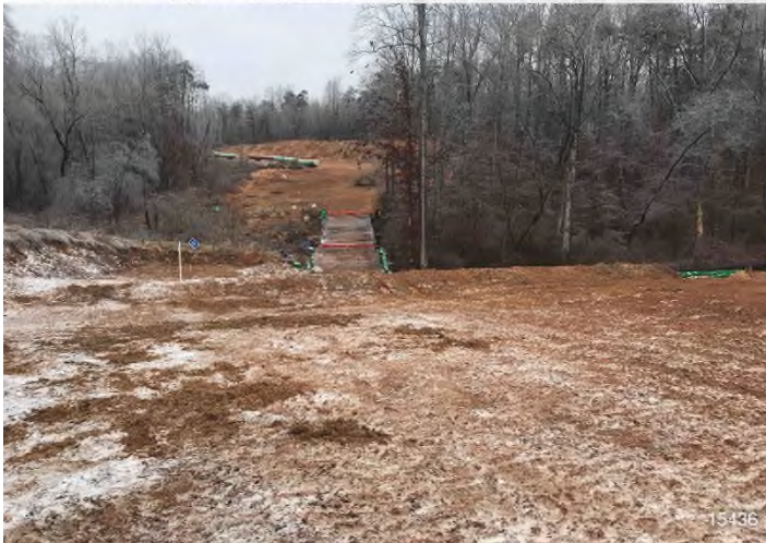
Figure 3: STA 15436+00 – Controls in place and functioning properly. Area stabilized with straw and erosion matting.
