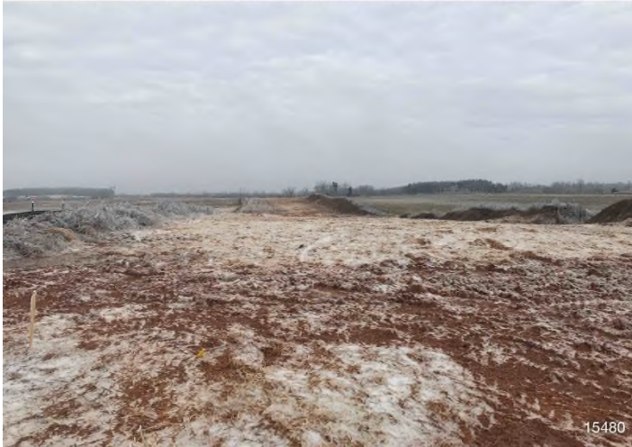
Figure 3: STA 15436+00 – Controls in place and functioning properly. Area stabilized with straw and erosion matting.
