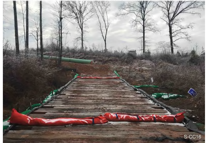
Figure 4: Stream S-CC16 – Controls in place and functioning properly around stream S-CC16.
