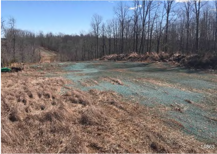
Figure 3: STA 14756+00 – Controls in place and functioning properly. Area stabilized with straw.
