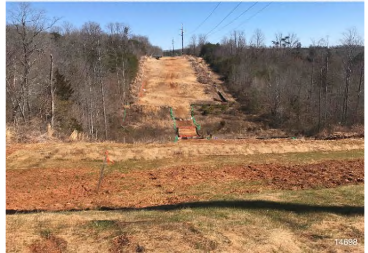
Figure 4: STA 14698+00 – Controls in place and functioning properly. Area stabilized with straw.
