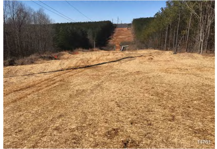
Figure 4: STA 14698+00 – Controls in place and functioning properly. Area stabilized with straw.
