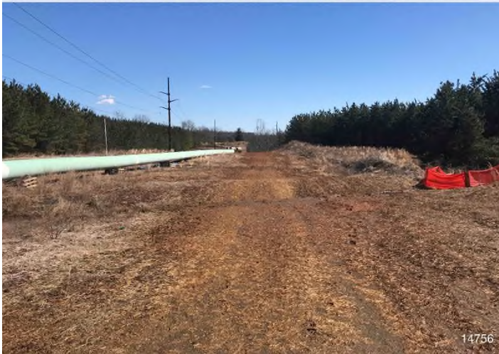
Figure 3: STA 14756+00 – Controls in place and functioning properly. Area stabilized with straw.
