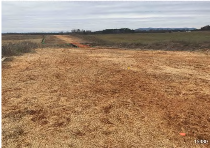
Figure 3: STA 13655+50 – Repair rill erosion and re-stabilization needed.
