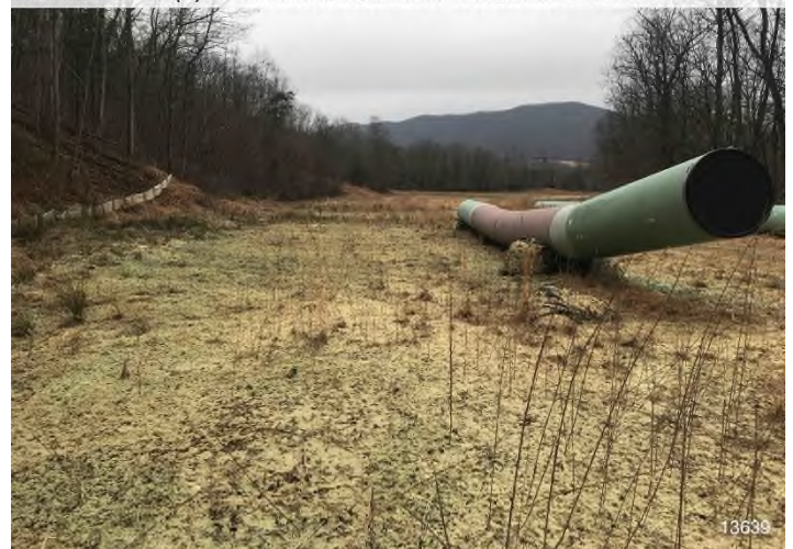
Figure 4: STA 13639+00 – Controls in place and functioning properly. Area stabilized with hydro-mulch.
