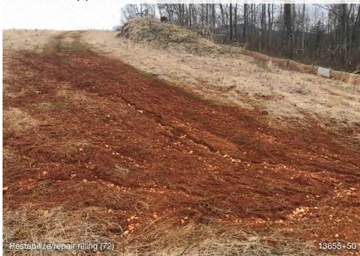
Figure 3: STA 13655+50 – Repair rill erosion and re-stabilization needed.
