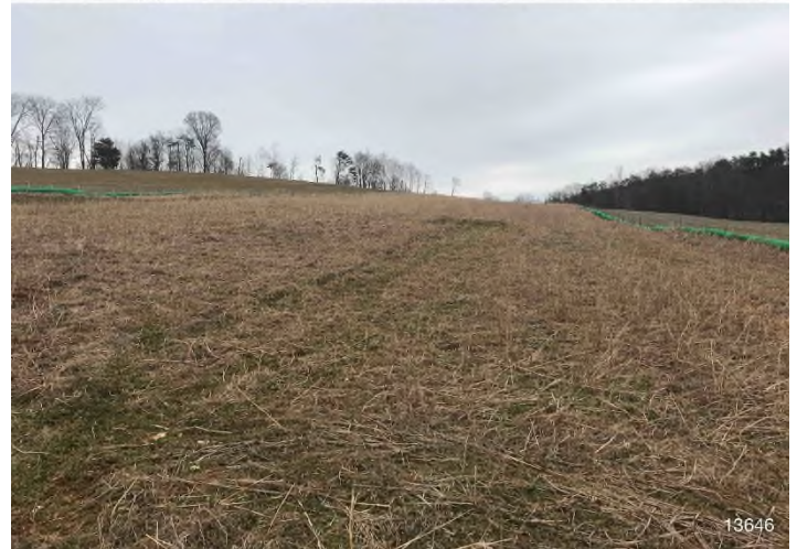
Figure 4: STA 13639+00 – Controls in place and functioning properly. Area stabilized with hydro-mulch.
