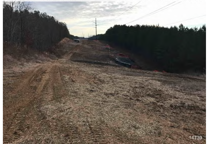
Figure 4: STA 14739+00 – Controls in place and functioning properly. Area stabilized with straw.
