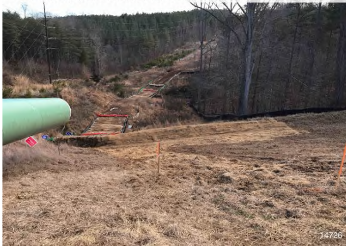
Figure 3: STA 14726+00 – Controls in place and functioning properly. Area stabilized with straw.
