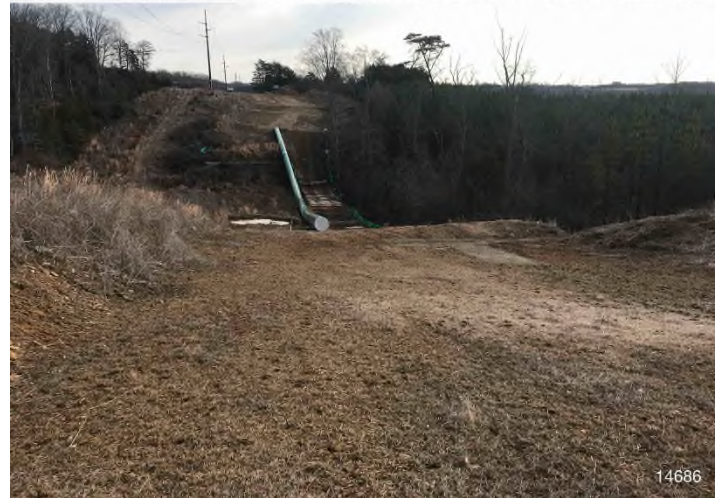
Figure 4: STA 14739+00 – Controls in place and functioning properly. Area stabilized with straw.
