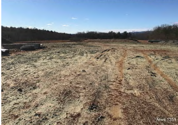
Figure 3: STA 13450+00 – Controls in place functioning properly. Area stabilized with straw.
