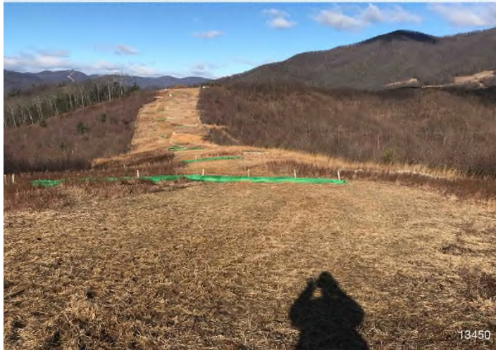
Figure 3: STA 13450+00 – Controls in place functioning properly. Area stabilized with straw.
