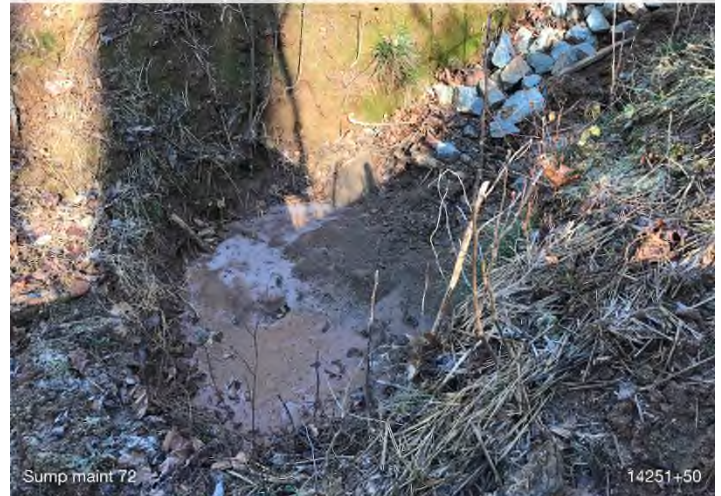
Figure 4: STA 14252+00 – Sump maintenance needed.
