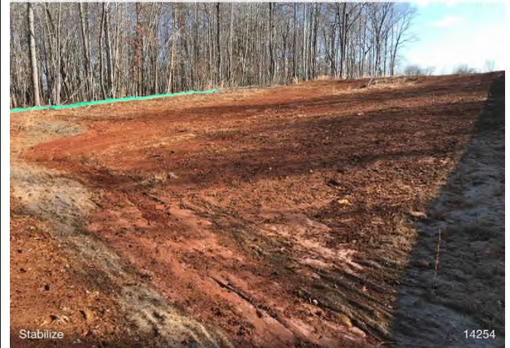
Figure 6: STA 14252+00 to 14256+00 – Re-stabilize ROW and stockpiles.
