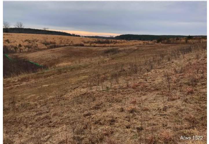
Figure 4: ATWS 1522 – Controls in place and functioning properly. Area stabilized with straw.
