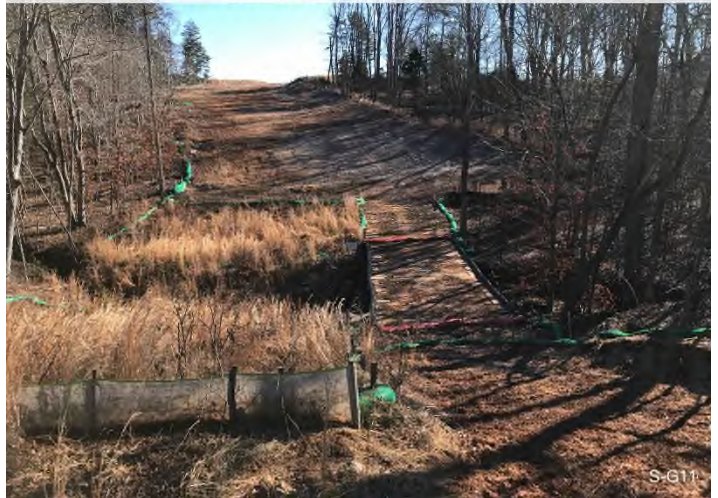
Figure 4: Stream S-G11 – Controls in place and functioning properly.
