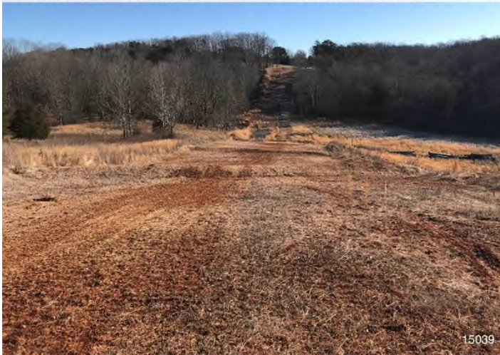
Figure 3: STA 15039+00 – Controls in place and functioning properly. Area stabilized with straw.
