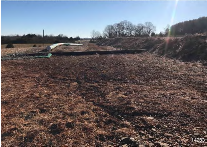
Figure 3: STA 15039+00 – Controls in place and functioning properly. Area stabilized with straw.
