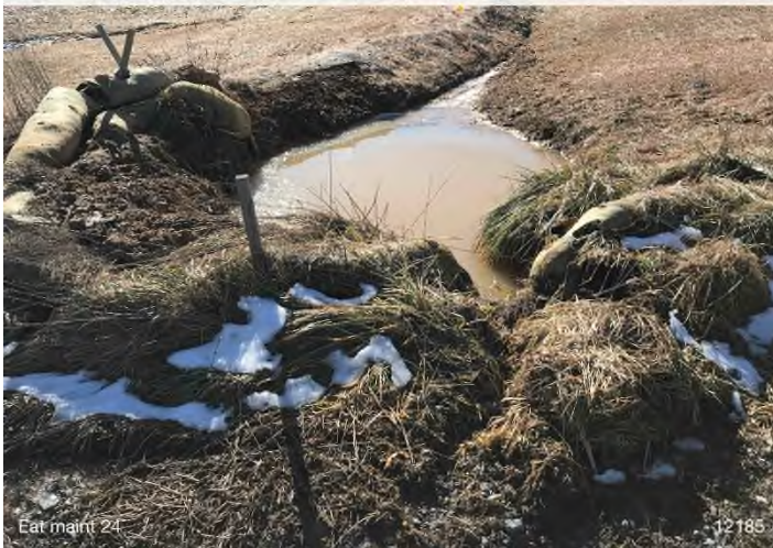
Figure 3: STA 12185+00 – End-treatment repair needed.
