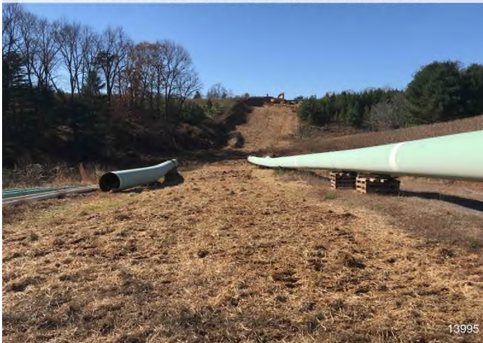
Figure 3: STA 13995+00 – Controls in place and functioning properly. Area stabilized with straw.
