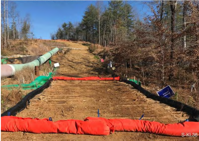
Figure 3: STA 13995+00 – Controls in place and functioning properly. Area stabilized with straw.
