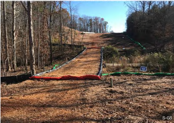
Figure 3: Stream S-G5 – Controls in place and functioning properly around S-G5 crossing. Area stabilized with straw.
