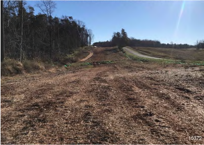
Figure 3: Stream S-G5 – Controls in place and functioning properly around S-G5 crossing. Area stabilized with straw.
