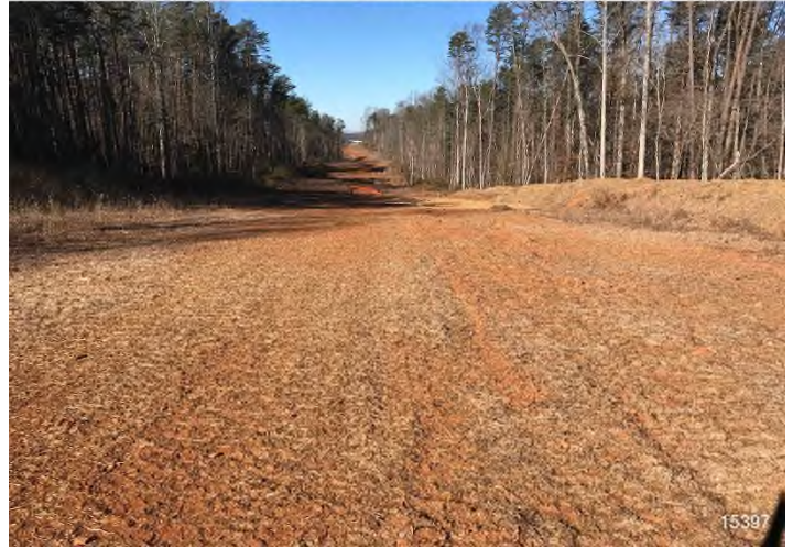
Figure 4: STA 15465+00 – Controls in place and functioning properly. Area stabilized with straw.
