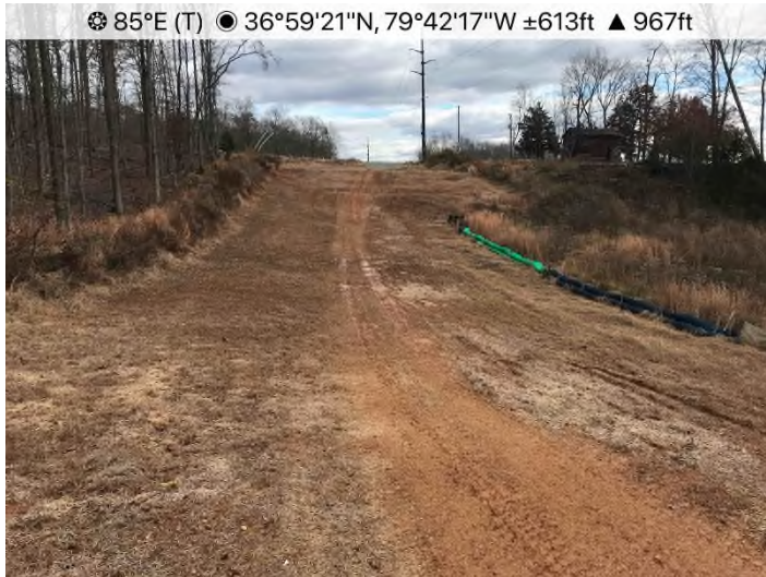
Figure 3: STA 14707+00 – Controls in place functioning properly. Area stabilized with straw.
