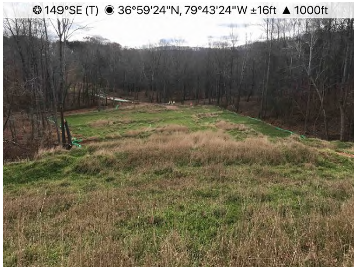
Figure 3: STA 14707+00 – Controls in place functioning properly. Area stabilized with straw.
