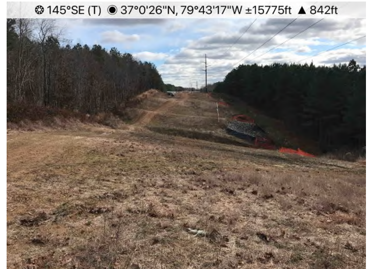
Figure 4: STA 14745+00 – Controls in place functioning properly. Area stabilized with straw.
