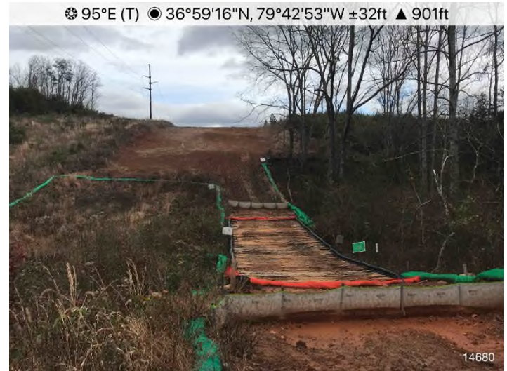
Figure 4: STA 14745+00 – Controls in place functioning properly. Area stabilized with straw.
