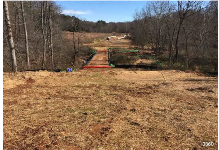
Figure 4: STA 13860+00 – Controls in place functioning properly. Area stabilized with straw.
