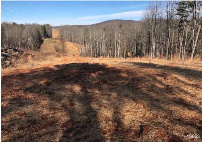
Figure 3: STA 13853+00 – Controls in place functioning properly. Area stabilized with straw.
