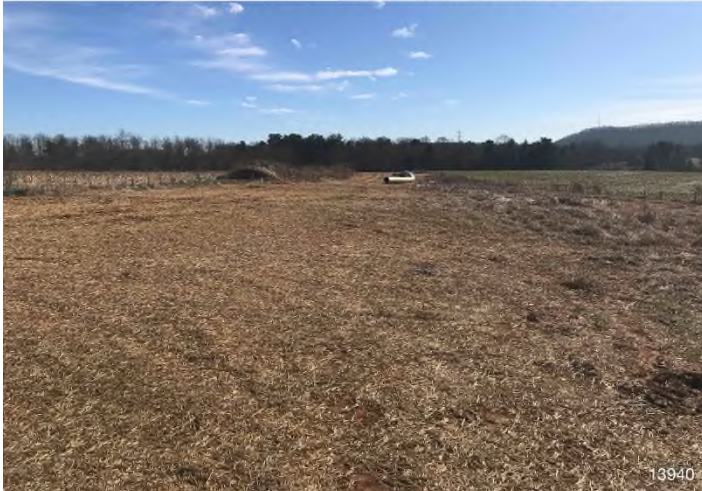
Figure 3: STA 13853+00 – Controls in place functioning properly. Area stabilized with straw.
