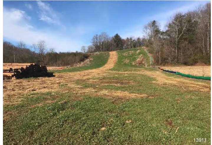
Figure 4: STA 13860+00 – Controls in place functioning properly. Area stabilized with straw.
