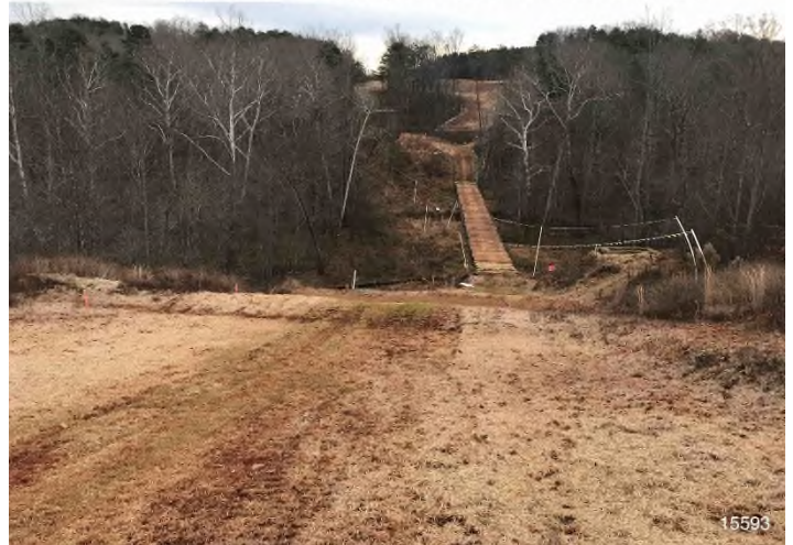
Figure 4: STA 15593+00 – Controls in place functioning properly. Area stabilized with straw.
