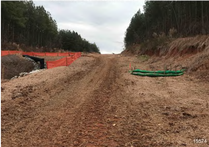
Figure 3: STA 15574+00 – Controls in place functioning properly. Area stabilized with straw.
