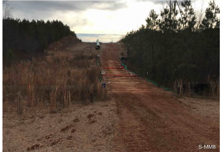
Figure 4: STA 15593+00 – Controls in place functioning properly. Area stabilized with straw.
