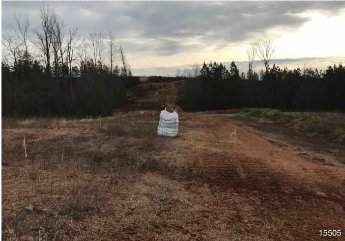
Figure 3: STA 15574+00 – Controls in place functioning properly. Area stabilized with straw.
