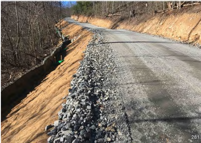
Figure 3: MVP-RO-281 – Controls in place and functioning properly. Contractor installing access road.
