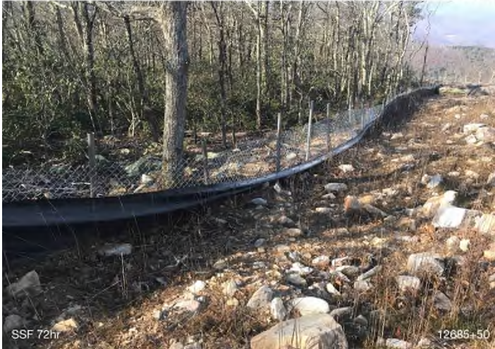
Figure 3: STA 12685+50 – SSF maintenance needed.
