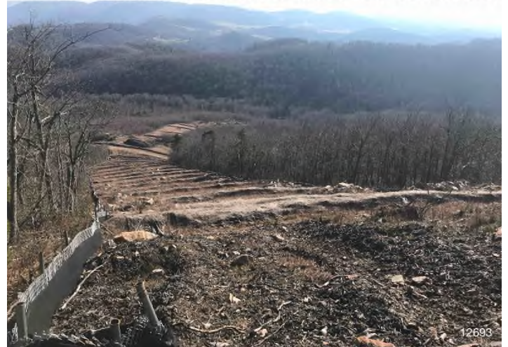
Figure 4: STA 12693+00 – Controls in place and functioning properly.
