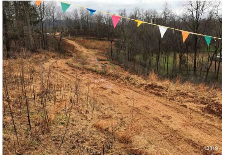
Figure 4: STA 13819+00 – Controls in place functioning properly. Area stabilized with straw.
