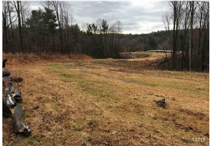
Figure 4: STA 13819+00 – Controls in place functioning properly. Area stabilized with straw.
