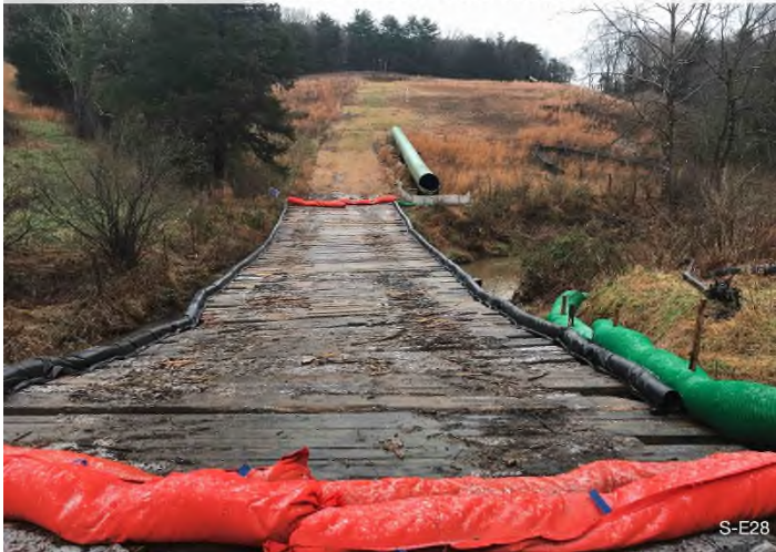
Figure 3: STA 13832+00 – Controls in place functioning properly. Area stabilized with straw.
