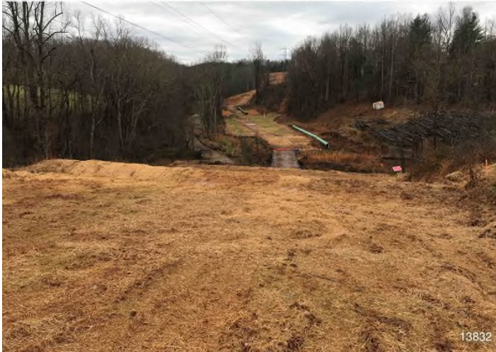
Figure 3: STA 13832+00 – Controls in place functioning properly. Area stabilized with straw.
