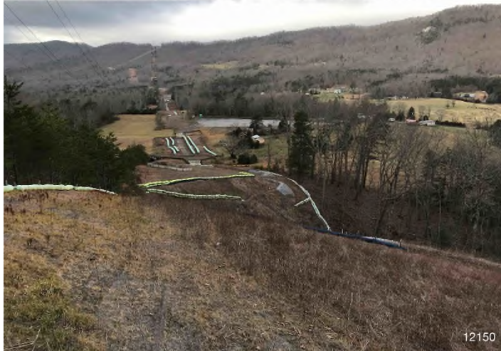
Figure 3: STA 12133+00 – Controls in place functioning properly. Area stabilized with straw.
