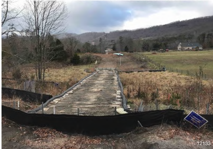
Figure 3: STA 12133+00 – Controls in place functioning properly. Area stabilized with straw.
