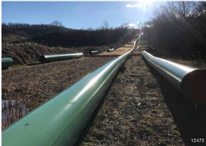
Figure 3: STA 12472+00 – Controls in place functioning properly. Area stabilized with straw and erosion matting.
