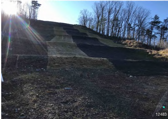
Figure 3: STA 12472+00 – Controls in place functioning properly. Area stabilized with straw and erosion matting.
