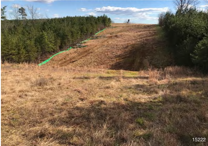
Figure 3: STA 14996+00 – Controls in place functioning properly. Area stabilized with straw.
