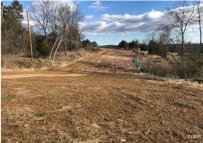
Figure 3: STA 14996+00 – Controls in place functioning properly. Area stabilized with straw.
