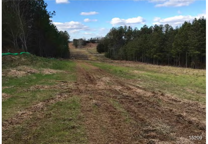
Figure 4: STA 15213+00 – Controls in place functioning properly. Area stabilized with straw.
