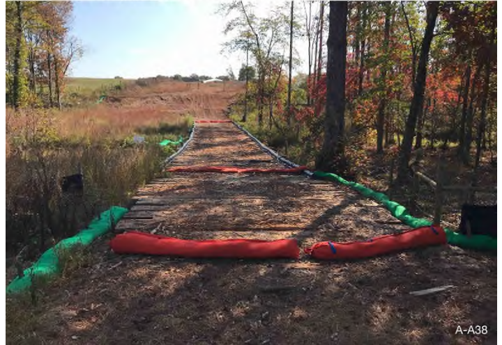
Figure 4: STRA 14385+00 – Controls in place and functioning properly. Area stabilized with straw.
