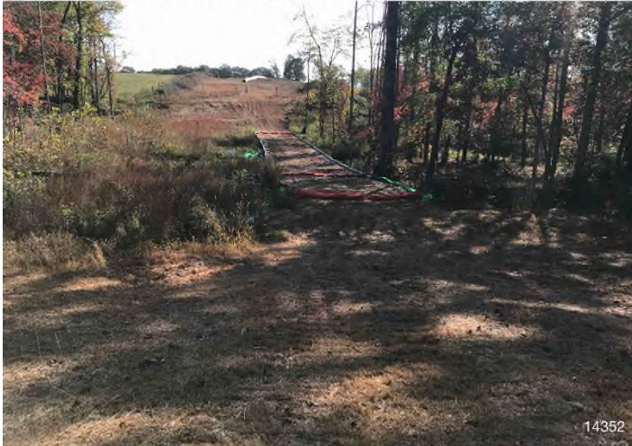
Figure 3: STRA 14360+00 – Controls in place and functioning properly. Area stabilized with straw.
