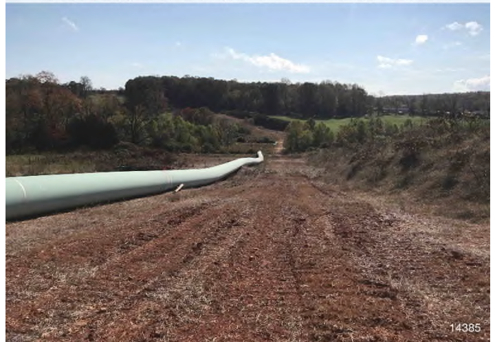
Figure 4: STRA 14385+00 – Controls in place and functioning properly. Area stabilized with straw.
