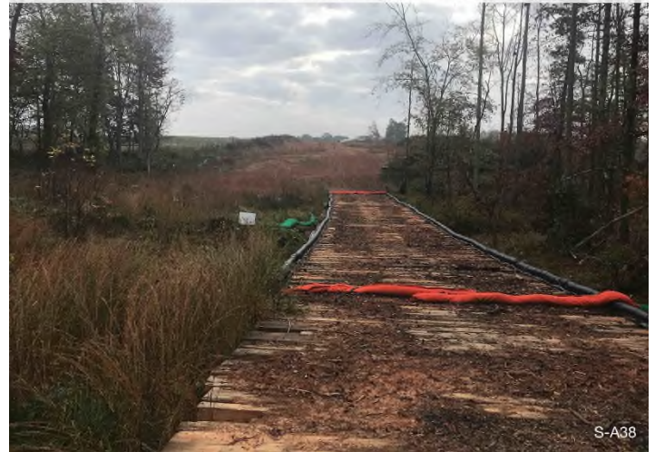
Figure 4: STA 14433+00 – Controls in place and functioning properly.
