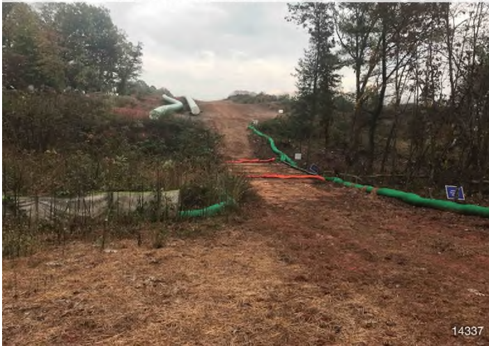
Figure 3: STA 14419+00 – Controls in place and functioning properly.
