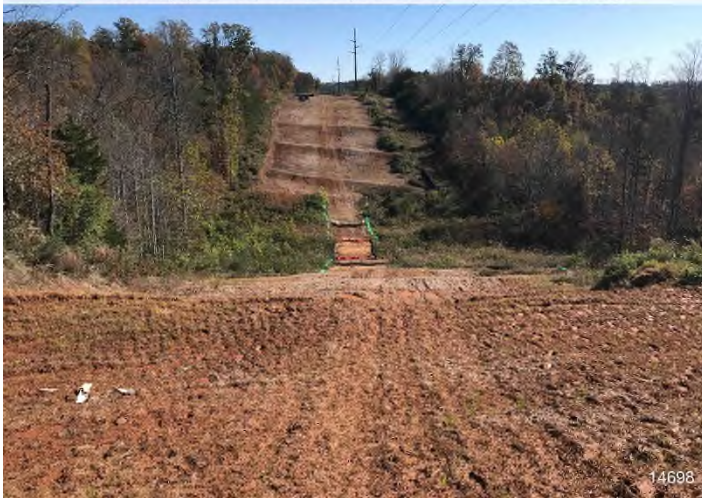
Figure 3: STA 14698+00 – Controls in place and functioning properly. Area stabilized with straw.
