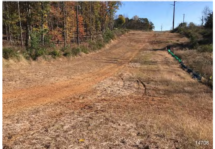
Figure 4: STA 14708+00 – Controls in place and functioning properly. Area stabilized with straw.
