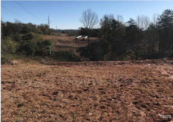
Figure 3: STA 14698+00 – Controls in place and functioning properly. Area stabilized with straw.
