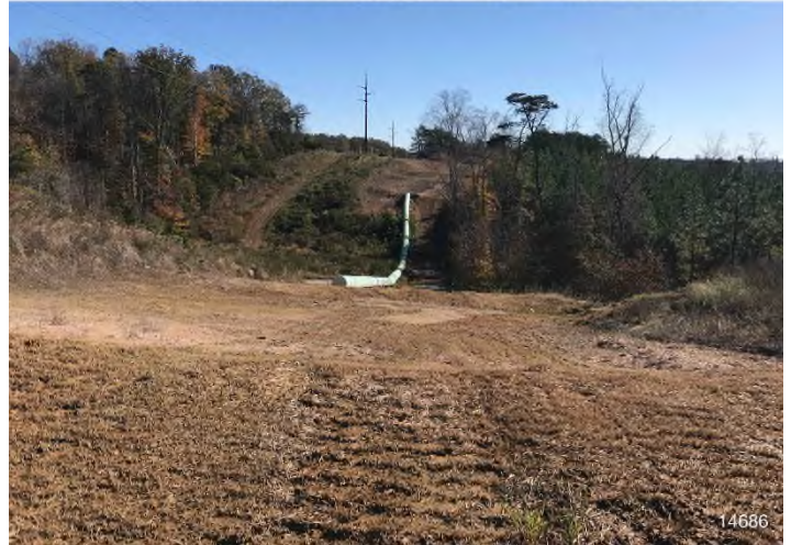
Figure 4: STA 14708+00 – Controls in place and functioning properly. Area stabilized with straw.
