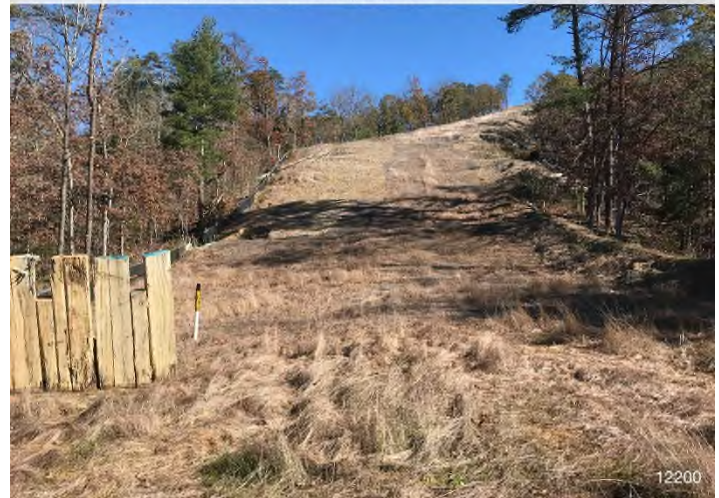
Figure 4: STA 12200+00 – Controls in place and functioning properly. Area stabilized with straw and erosion matting.
