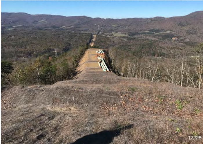
Figure 3: STA 12212+00 – Controls in place and functioning properly. Area stabilized with straw and erosion matting.
