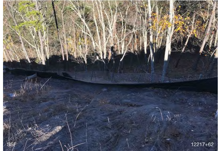
Figure 4: STA 12200+00 – Controls in place and functioning properly. Area stabilized with straw and erosion matting.
