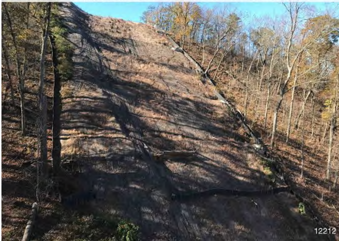
Figure 3: STA 12212+00 – Controls in place and functioning properly. Area stabilized with straw and erosion matting.
