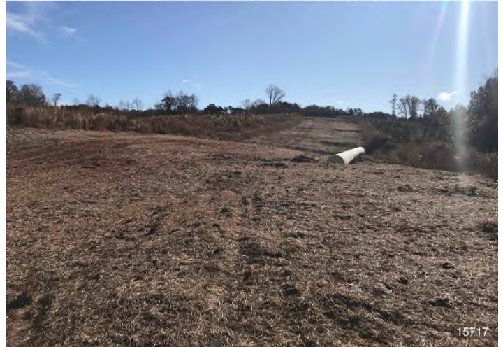
Figure 4: STA 15815+00 – Controls in place and functioning properly. Area stabilized with straw.
