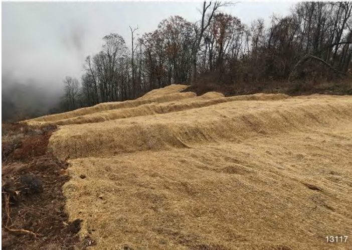
Figure 3: STA 12965+00 – Contractor stripping topsoil and building temp. waterbars. Perimeter controls in place.
