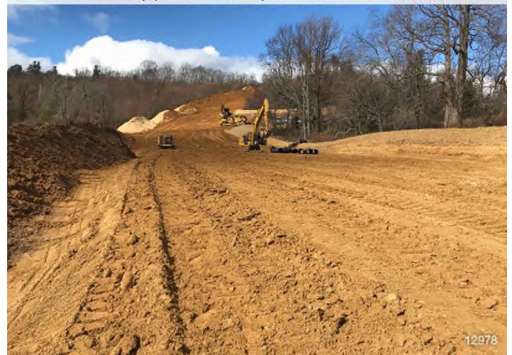
Figure 4: STA 12978+00 – Contractor installing Clean Water Diversion pipe and stabilizing stockpiles.
