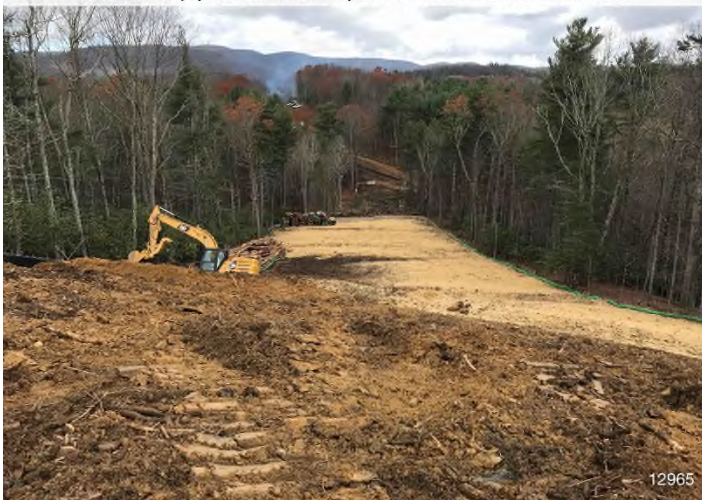
Figure 3: STA 12965+00 – Contractor stripping topsoil and building temp. waterbars. Perimeter controls in place.
