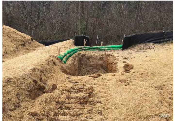
Figure 4: STA 12978+00 – Contractor installing Clean Water Diversion pipe and stabilizing stockpiles.
