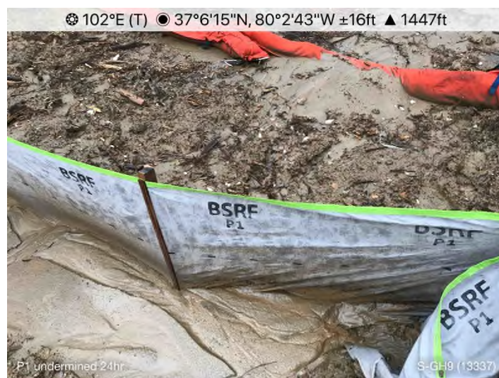
Figure 3: STA 13337+00 – P1 undermined.
