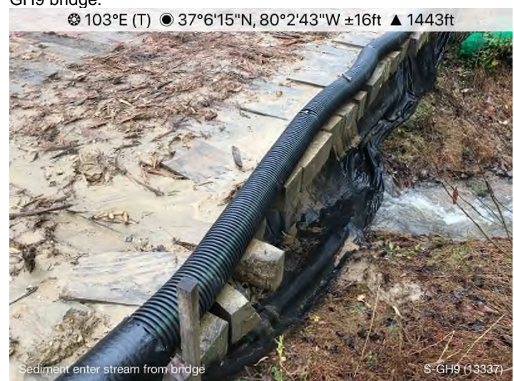
Figure 4: STA 13337+00 – Sediment impacting stream from S-GH9 bridge.
