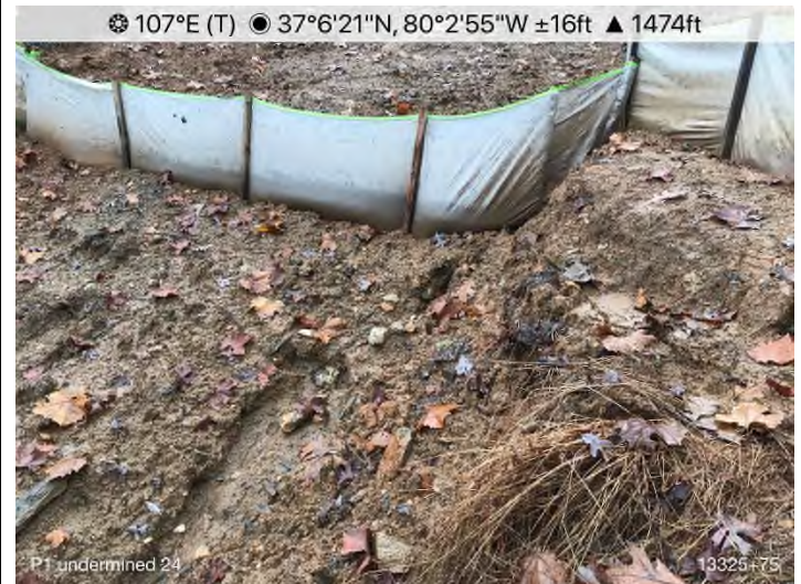
Figure 12: STA 13325+75 – P1 undermined.
