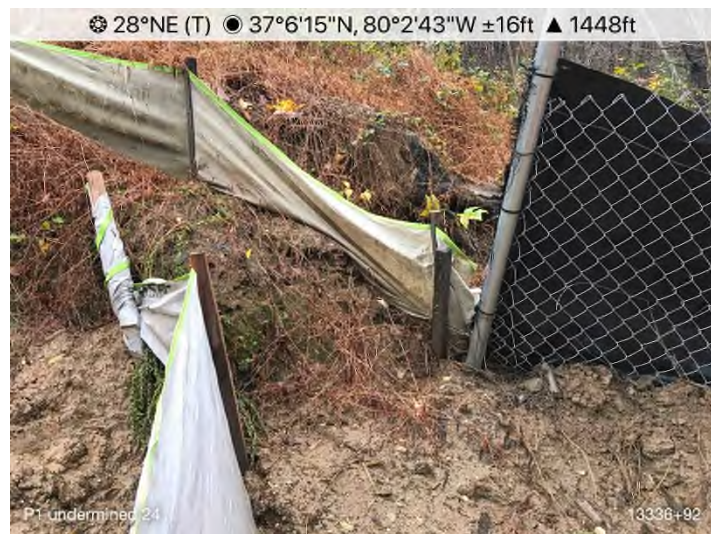
Figure 7: STA 13333+59 – Sump cleanout needed.
