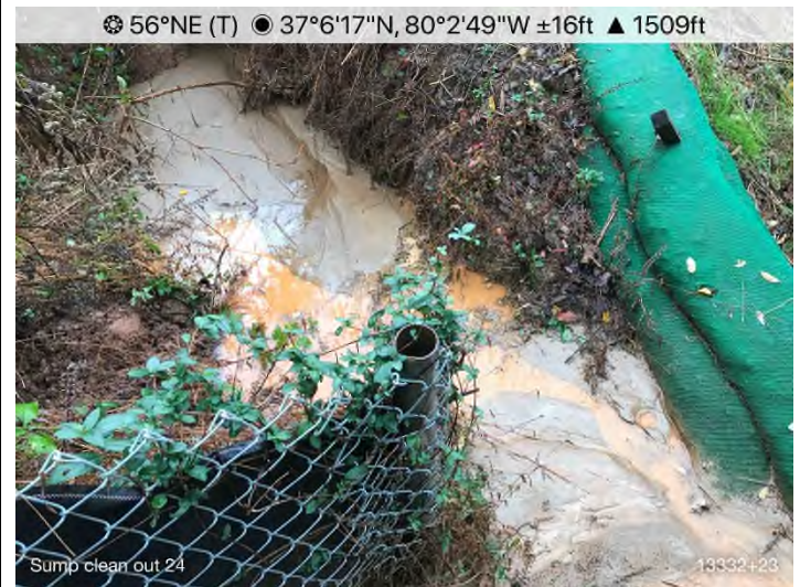
Figure 12: STA 13325+75 – P1 undermined.
