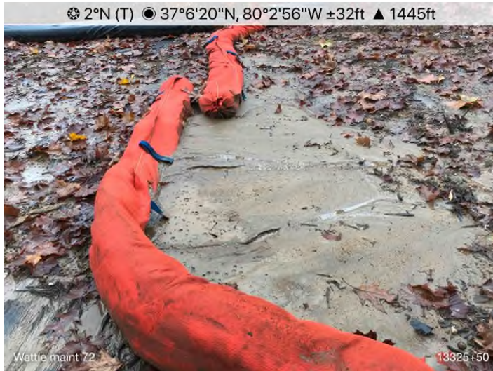
Figure 13: STA 13325+50 – Stream S-GH11 bridge wattle cleanout needed.
