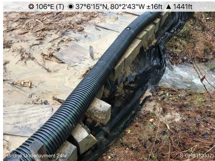
Figure 3: STA 13337+00 – P1 undermined.
