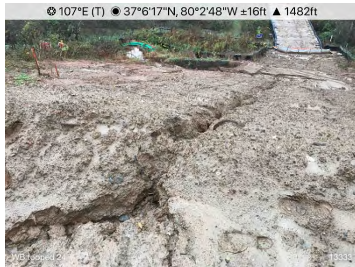
Figure 11: STA 13332+33 – Sediment discharged off ROW from sump at STA 13332+23.
