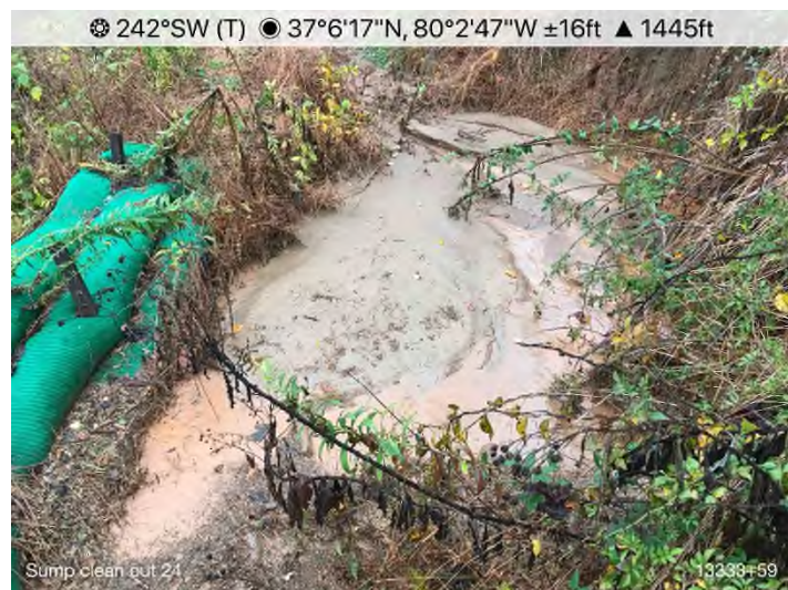
Figure 7: STA 13333+59 – Sump cleanout needed.
