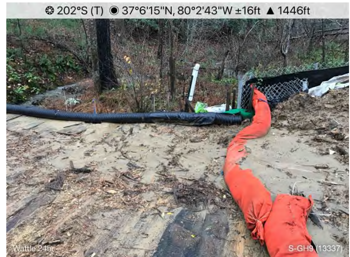
Figure 4: STA 13337+00 – Sediment impacting stream from S-GH9 bridge.
