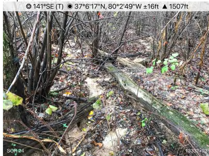
Figure 11: STA 13332+33 – Sediment discharged off ROW from sump at STA 13332+23.
