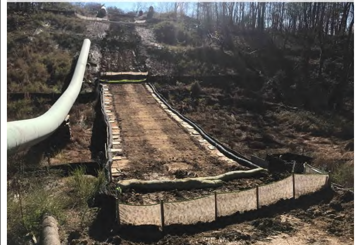
Figure 4: STA 13331+00 – Controls in place and functioning properly. Travel lane active and disturbed
