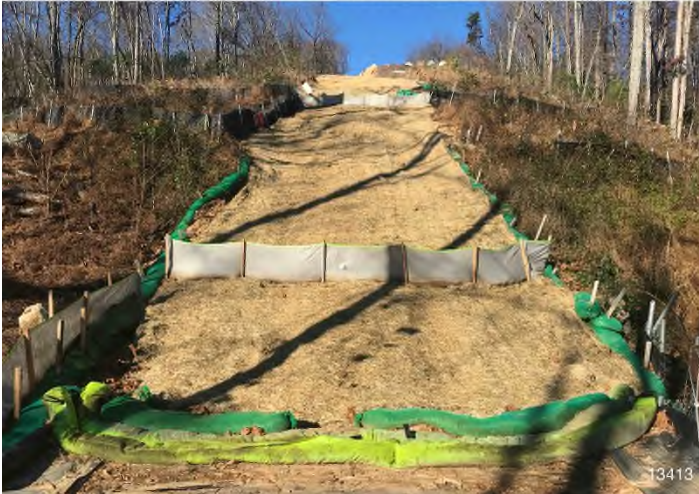
Figure 3: STA 13385+00 – Controls in place and functioning properly. Travel lane active and disturbed.
