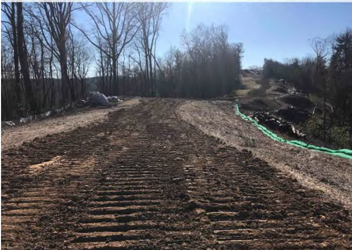
Figure 3: STA 13385+00 – Controls in place and functioning properly. Travel lane active and disturbed.
