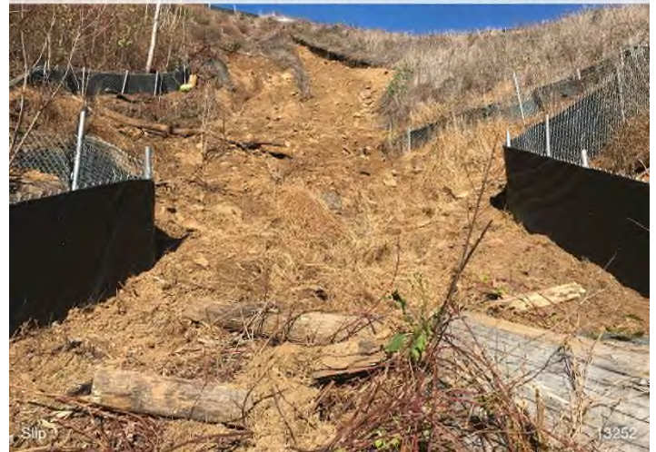
Figure 4: STA 13252+00 – Looking northwest toward the slope failure. SSF perimeter installed around the area.
