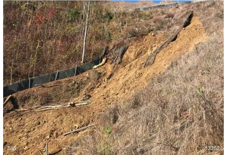
Figure 4: STA 13252+00 – Looking northwest toward the slope failure. SSF perimeter installed around the area.
