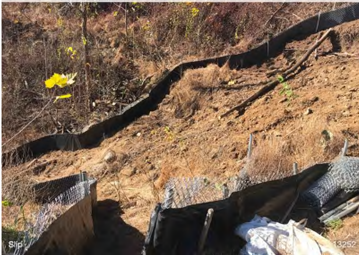
Figure 3: STA 13252+00 – Looking southwest at the slip area from within the ROW. SSF perimeter installed around the area.
