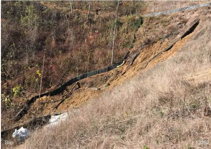
Figure 3: STA 13252+00 – Looking southwest at the slip area from within the ROW. SSF perimeter installed around the area.
