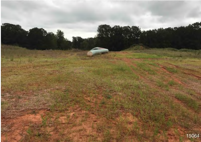
Figure 3: STA 15081+00 – Controls in place and functioning properly. Area stabilized with straw.
