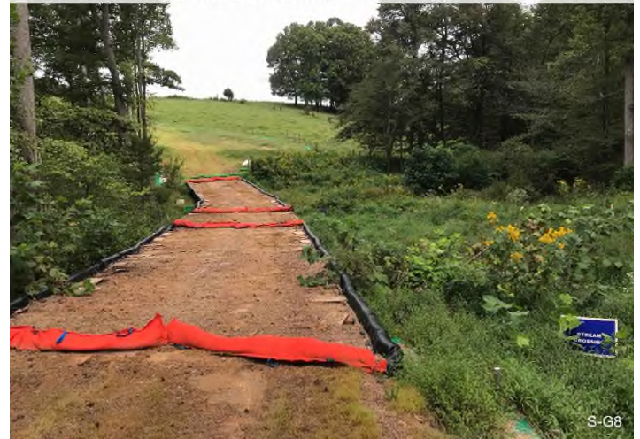
Figure 4: Stream S-G8 – Controls in place and functioning properly around stream S-G8 crossing.
