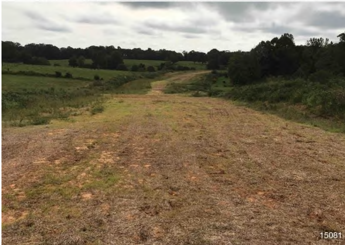
Figure 3: STA 15081+00 – Controls in place and functioning properly. Area stabilized with straw.
