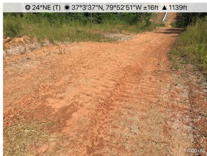
Figure 3: STA 14030+00 – Re-stabilization needed.
