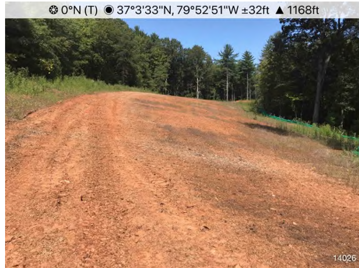
Figure 3: STA 14030+00 – Re-stabilization needed.
