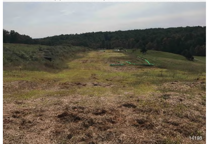
Figure 4: STA 14198+00 – Controls in place and functioning properly. Area stabilized with straw.
