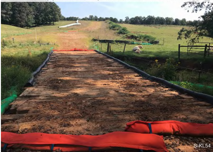
Figure 3: Stream S-KL54 – Controls in place and functioning properly around S-KL54 crossing.
