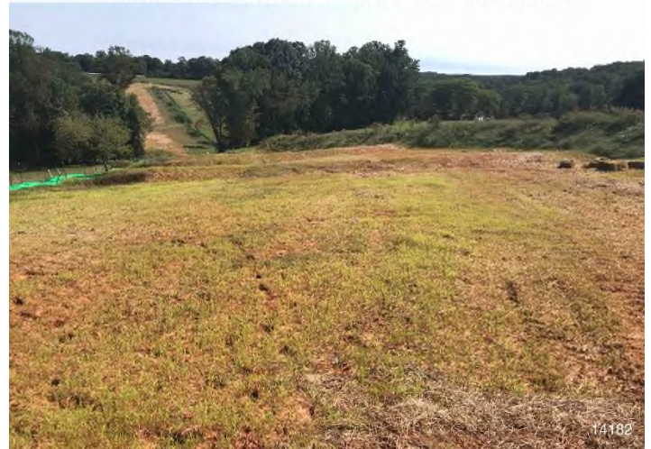
Figure 4: STA 14198+00 – Controls in place and functioning properly. Area stabilized with straw.
