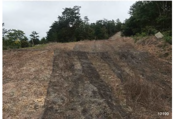
Figure 4: STA 12210+00 – Controls in place and functioning properly. Area stabilized with straw and erosion matting.
