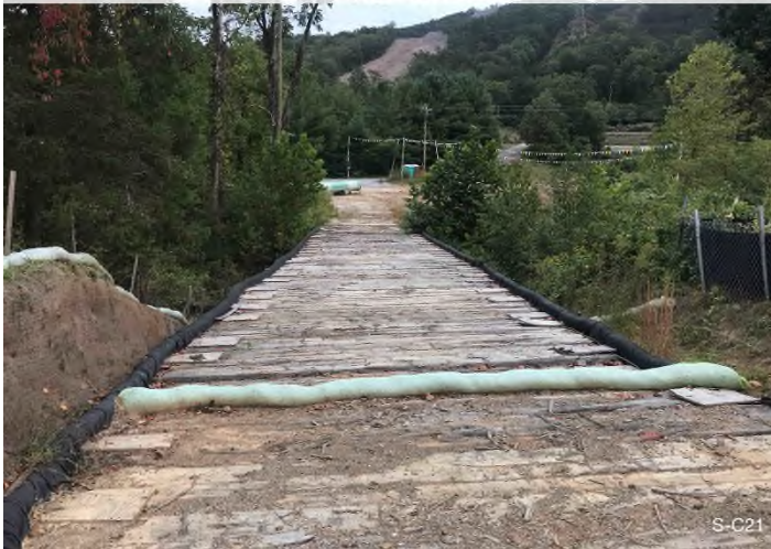
Figure 3: STA 12200+00 – Controls in place and functioning properly. Area stabilized with straw and erosion matting.
