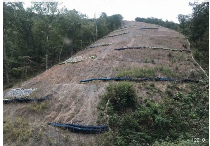
Figure 4: STA 12210+00 – Controls in place and functioning properly. Area stabilized with straw and erosion matting.
