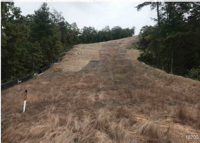
Figure 3: STA 12200+00 – Controls in place and functioning properly. Area stabilized with straw and erosion matting.
