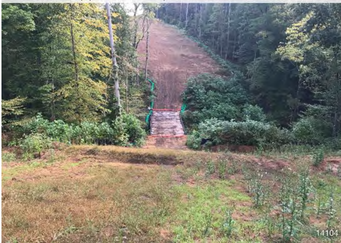
Figure 3: STA 14104+00 – Controls in place and functioning properly. Area stabilized with straw and erosion matting.
