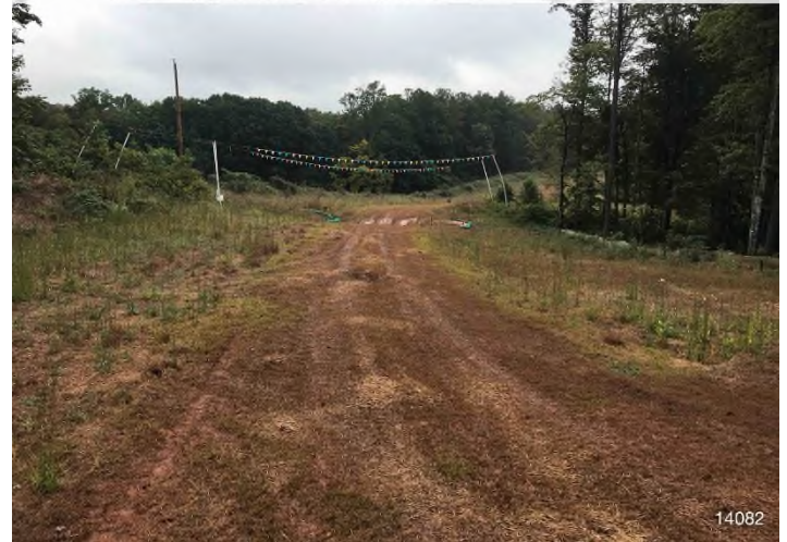
Figure 4: STA 14155+00 – Controls in place and functioning properly. Area stabilized with straw and erosion matting.
