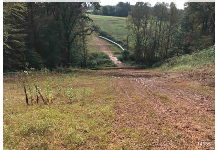
Figure 4: STA 14155+00 – Controls in place and functioning properly. Area stabilized with straw and erosion matting.
