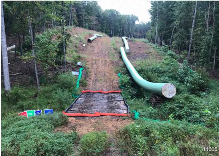
Figure 3: STA 14104+00 – Controls in place and functioning properly. Area stabilized with straw and erosion matting.
