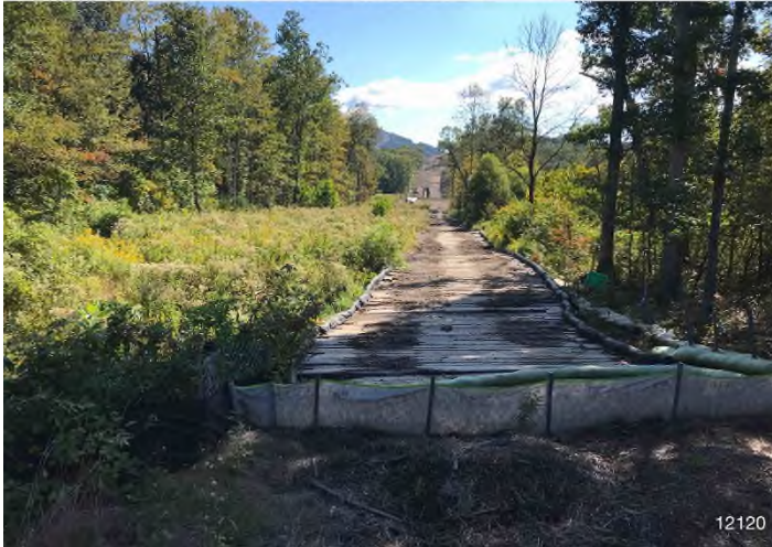
Figure 3: STA 12188+00 – Controls in place and functioning properly. Area stabilized with straw.
