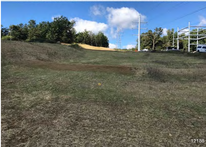
Figure 3: STA 12188+00 – Controls in place and functioning properly. Area stabilized with straw.
