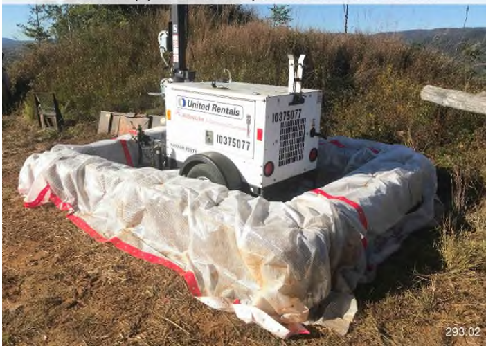
Figure 3: MVP-FR-293.02 – Secondary containment in place and functioning properly.
