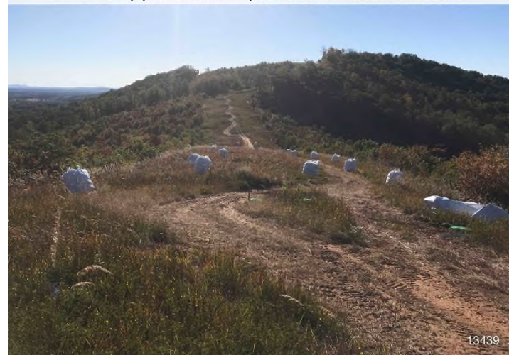
Figure 4: STA 13439+00 – PPL actively working to replace CFS in area.
