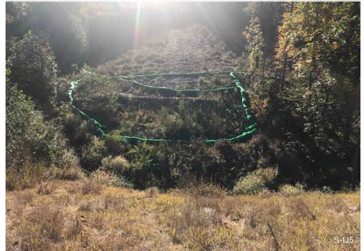
Figure 4: STA 13439+00 – PPL actively working to replace CFS in area.
