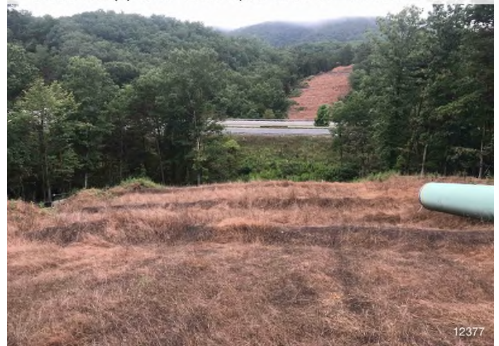
Figure 4: STA 12377+00 – Controls in place and functioning properly. Area stabilized with erosion matting and straw.
