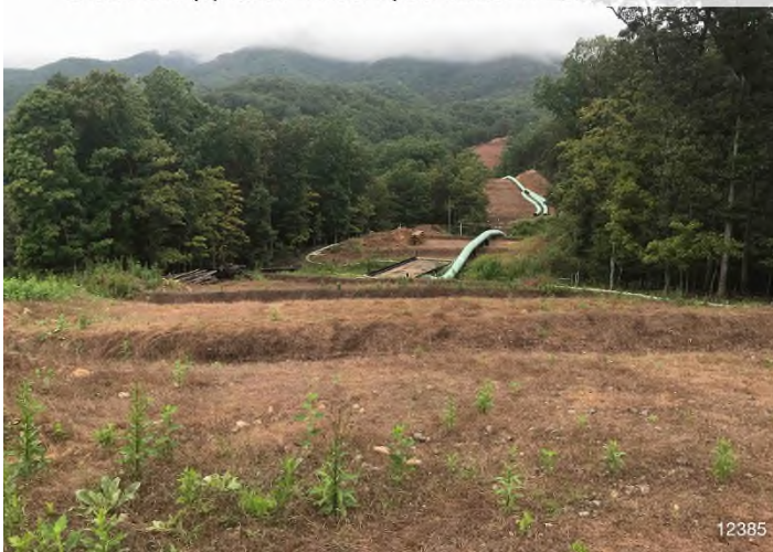
Figure 3: STA 12385+00 – Controls in place and functioning properly. Area stabilized with erosion matting and straw.
