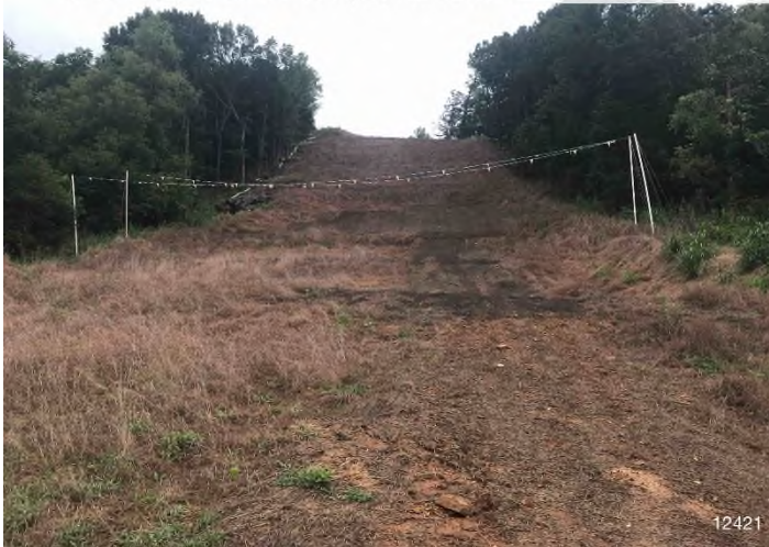
Figure 3: STA 12385+00 – Controls in place and functioning properly. Area stabilized with erosion matting and straw.
