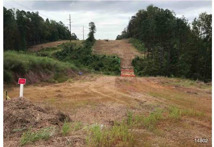
Figure 4: STA 14815+75 – Unauthorized offsite LDA impacting perimeter MVP controls. Controls being repaired.
