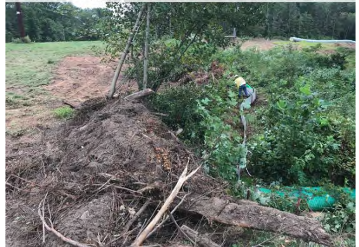
Figure 4: STA 14815+75 – Unauthorized offsite LDA impacting perimeter MVP controls. Controls being repaired.
