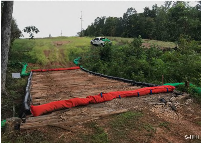
Figure 3: Stream S-HH1 – Controls in place and functioning properly around stream S-HH1 crossing.
