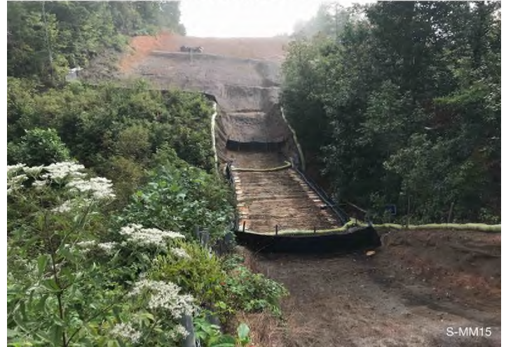
Figure 4: STA 12116+00 – Controls in place and functioning properly.
