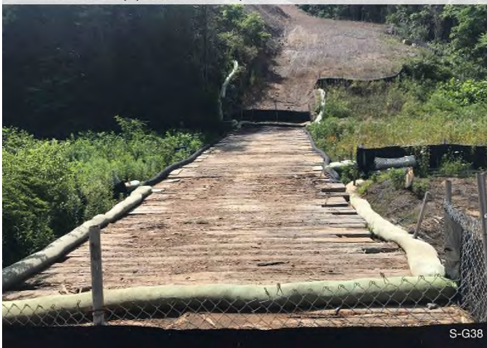
Figure 3: Stream S-G38 – Controls in place and functioning properly around stream crossing.
