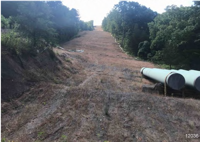
Figure 3: Stream S-G38 – Controls in place and functioning properly around stream crossing.
