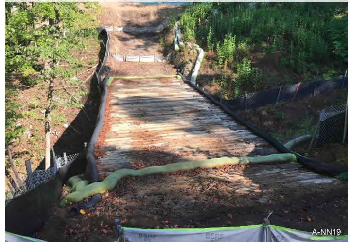
Figure 4: Stream S-NN19 – Controls in place and functioning properly around stream crossing.
