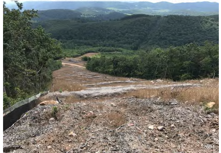
Figure 4: STA 12694+00 – Controls in place and functioning properly. Area stabilized with erosion matting and Earth Guard.
