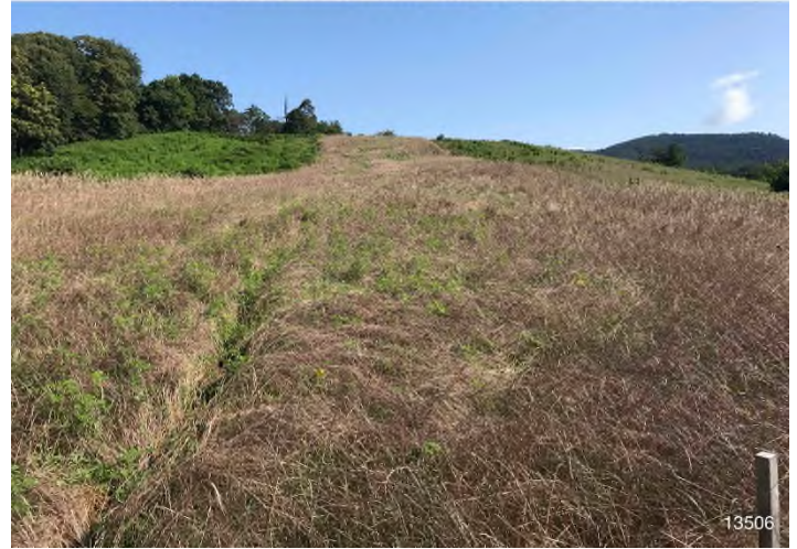
Figure 4: STA 12694+00 – Controls in place and functioning properly. Area stabilized with erosion matting and Earth Guard.
