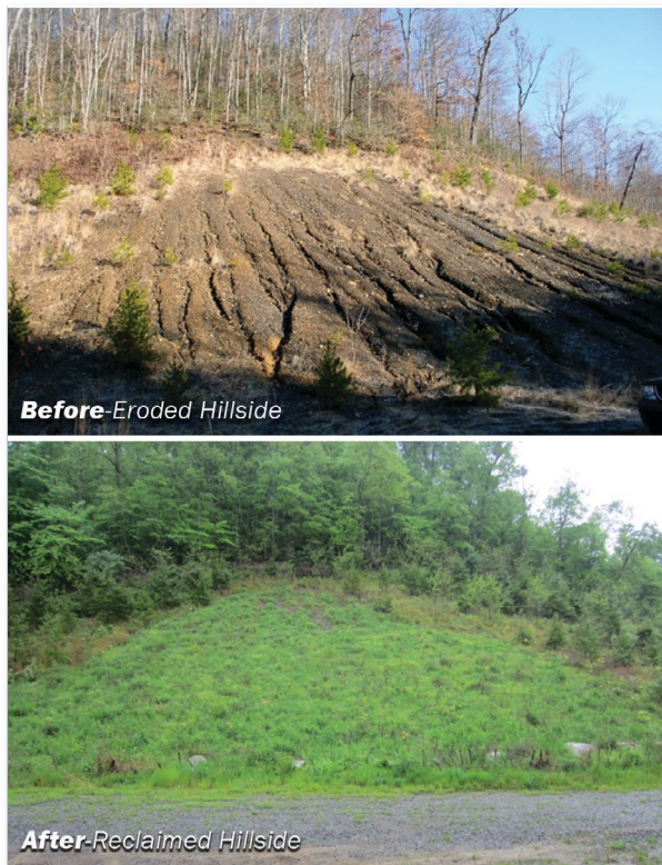
Figure 2. Before and after reclaiming a hillside at the Gilbert site in the Stone Creek watershed.
