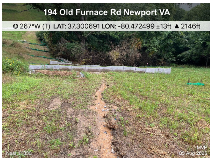
Fig. 3 Near STA 11330: rill erosion has occurred.
