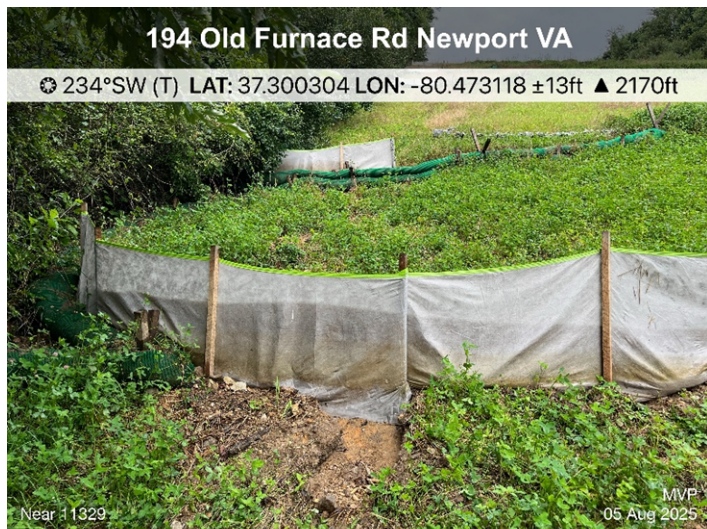
Fig. 1 Near STA 11329: P1 is undermined.
