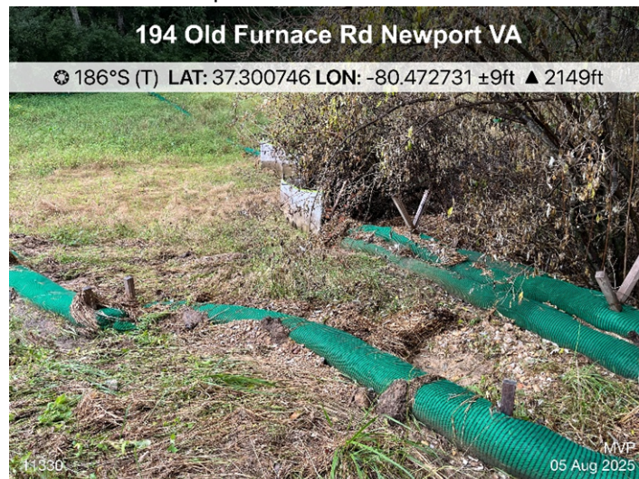
Fig. 2 STA 11330: CFS requires maintenance.
