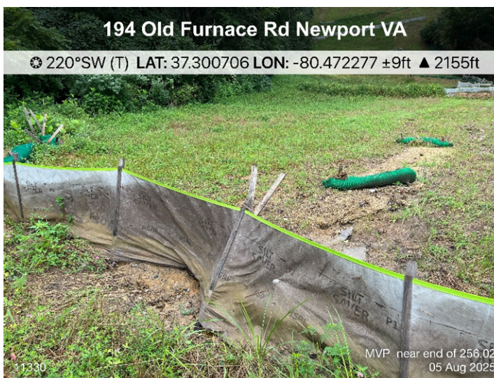
Fig. 4 STA 11330: P1 is undermined.
