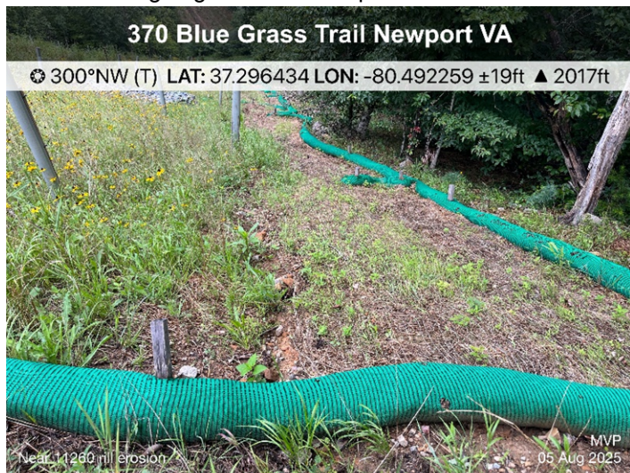
Fig. 9 STA 10816: ongoing installation of permanent waterbars.
