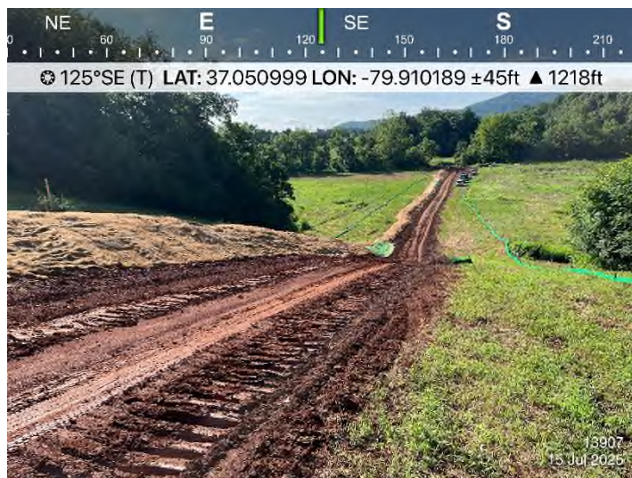
Figure 2: STA 13907+00 – Travel lane installed for access to S-II2 bank repair. Controls in place and functioning properly.
